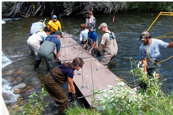
PIT-tag antennae being installed in Lemhi River, Idaho.
